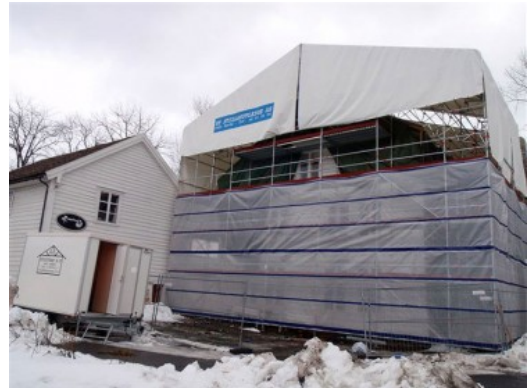
Figure 6.1-2 Scaffolding cover- (Axelsson, 2004).
